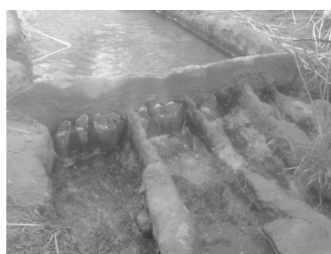
Fig. no. 4. An example of a kasria in the southwest of Algeria [6]
