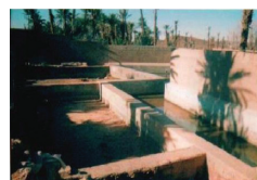
Fig. no. 5. The water storage basin "Majen", January 2008
