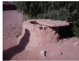
Fig. no. 3. A well foggara in the oasis of Lahmar, in January 2008
