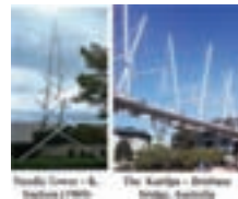
Figure 14 Structures that use tensegrity systems
